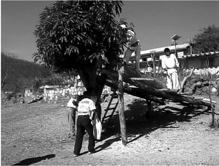
Figure 6.6. Carpentry at the CETMK.
